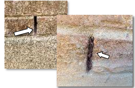
Item F (weep hole with & without mesh)
