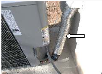
Item E (sample photo of UV protection)
