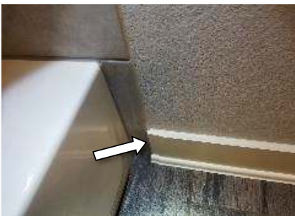
Item A (sample photo of caulking location)
