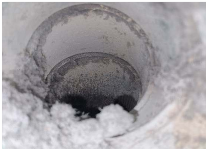
View inside dryer vent (OK)
