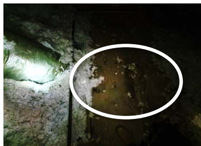
Item M (below furnace flue)
