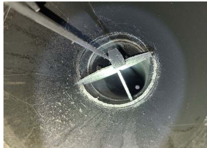
View up fireplace flue (OK)
