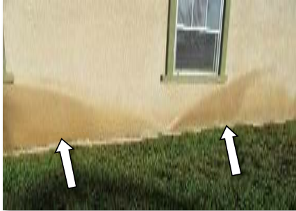
Item C (sample photo of head spraying wall)
