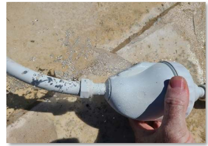
Photo of robot reversing valve operating
