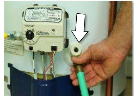
Item A (where to attach drain hose)
